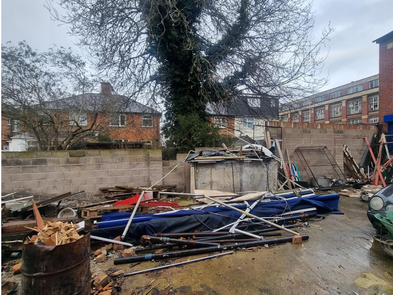
View of rear of Marina Road properties
