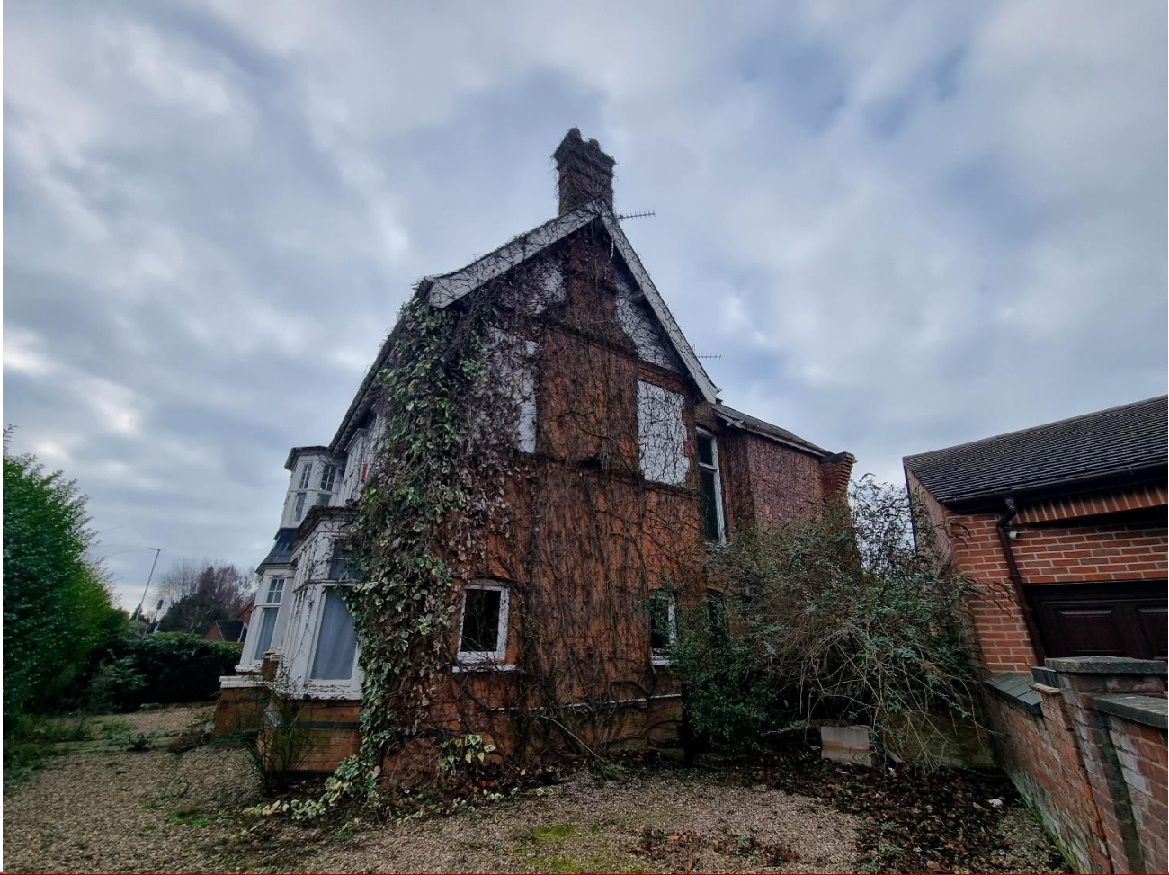
View of north elevation
