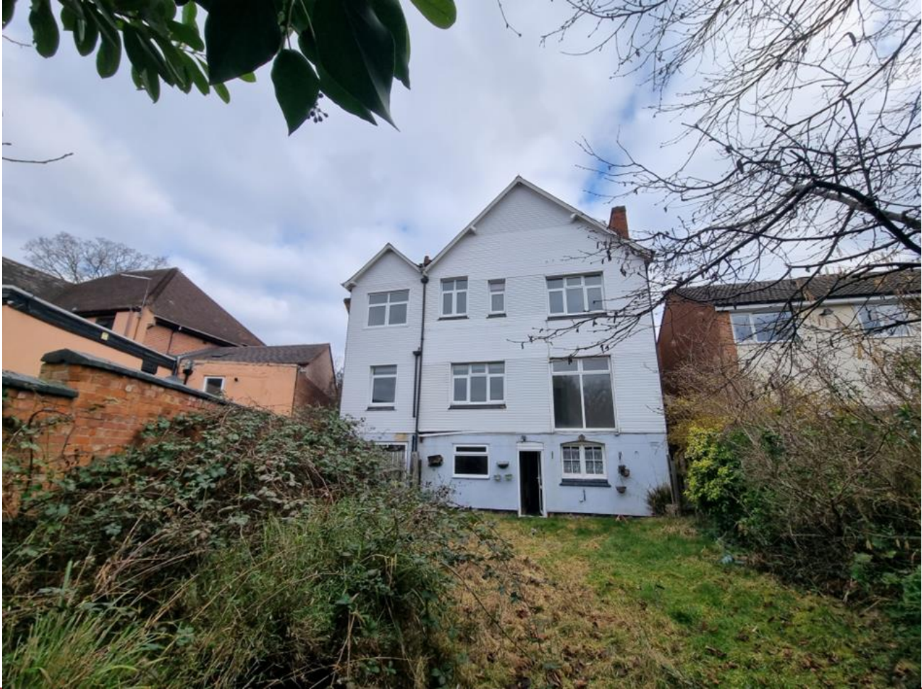
View of rear elevation
